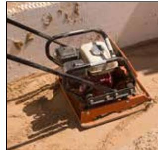
Backfill should also be compacted properly. Fill should be placed about 2 feet or less in depth, beginning with gravel, transitioning to soil, using a small compacting machine to compress the soil evenly around the foundation. **DO NOT use a tractor to compact the soil all at once after filling.** This can cause damage to the waterproofing
