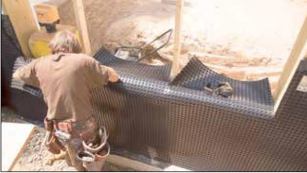
DMX AG membrane attached below large opening.
