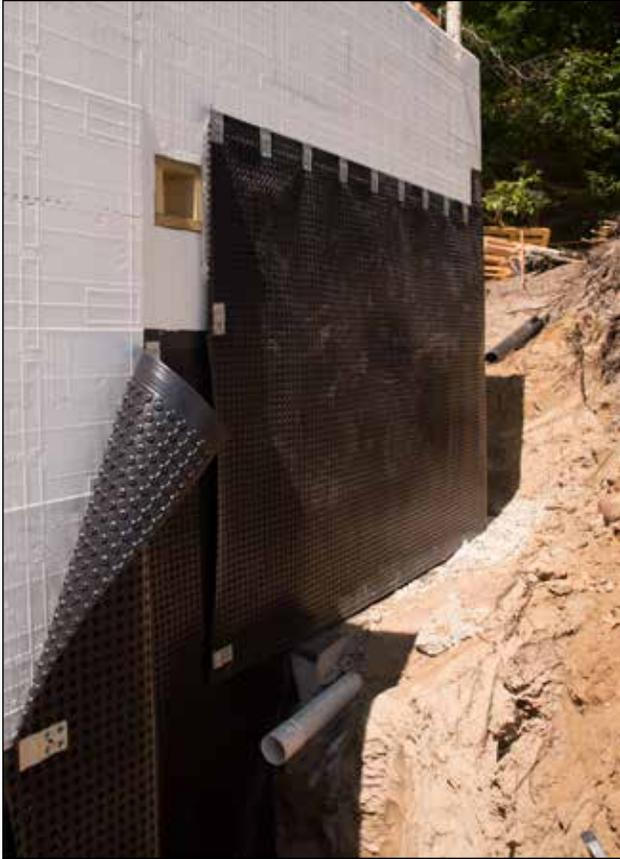
Waterproofing membrane and air gap membranes installed and mechanically attached above grade levels.
