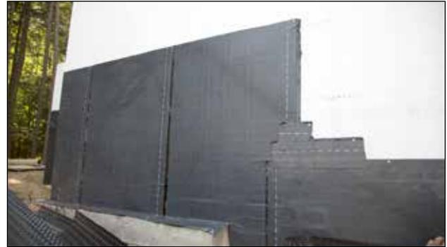
Adhesive waterproofing membrane installed. Note overlap on all seams and mechanical attachment at the top of the membrane.
