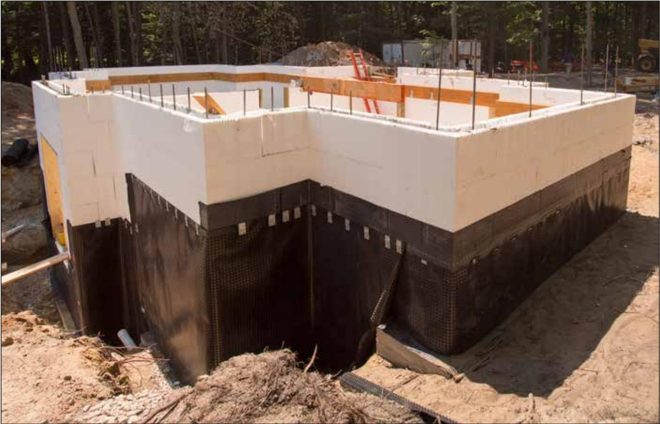
Typical walkout ICF basement using a waterproofing barrier and an air gap membrane installed as well as perimeter foundation drainage.
